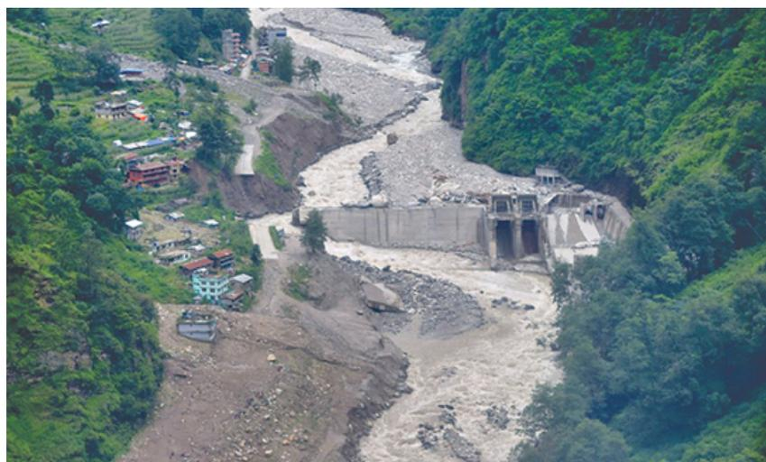
**Figure 2:** Damaged dam of the Upper Bhotekoshi Hydropower Project after flooding on 5 July 2016 on the Bhotekoshi River in Sindhupalchowk district, Nepal [18].
